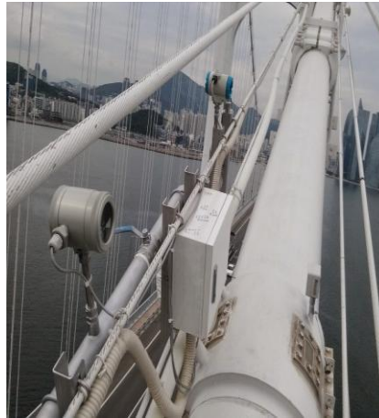
Busan Gwangandaegyo & Yeongjong Bridge Cable air-insert valve type 22 units delivered
